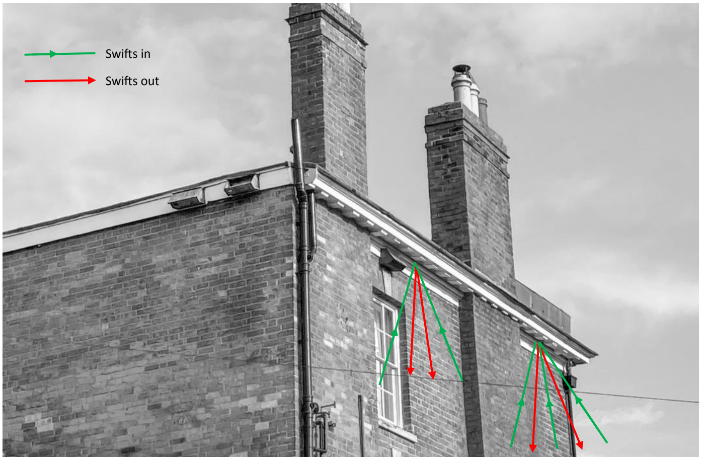
A house in The Southend. 7th July 2023
